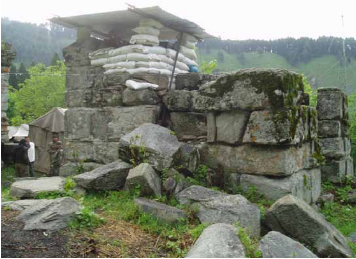
Photo 3: 2000 Year old Hindu temple made from Panjal traps flood basalt. Now being used as a military outpost.
